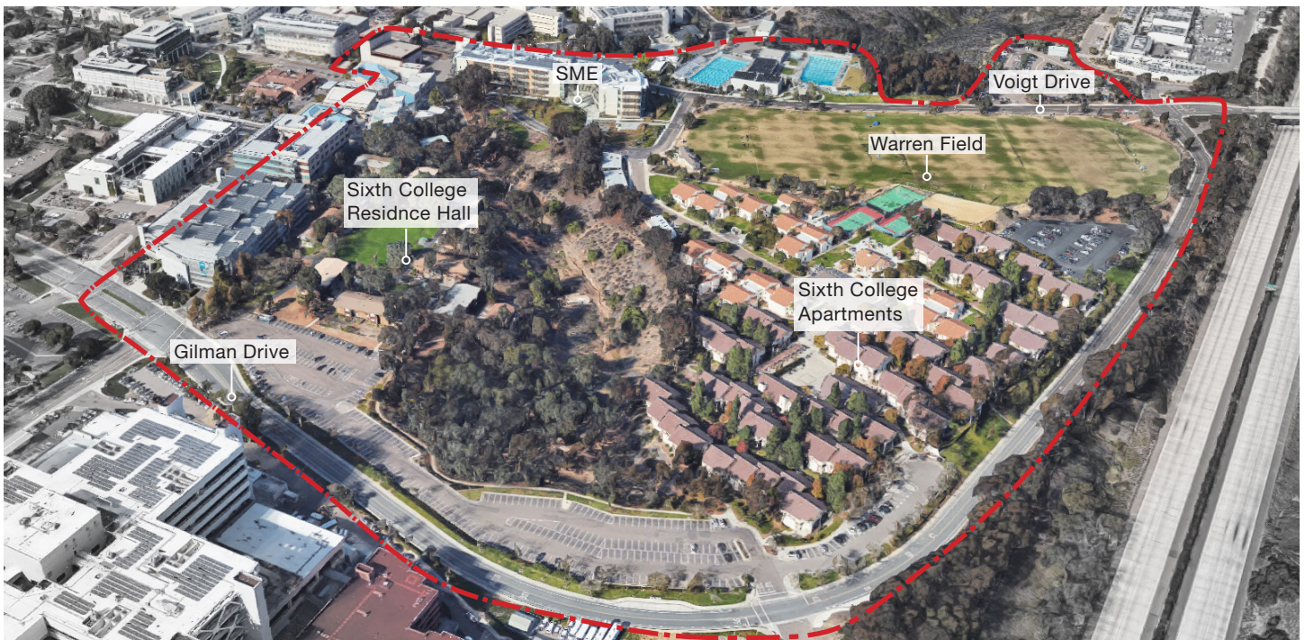
Pepper Canyon Neighborhood Prior to Light Rail Construction
