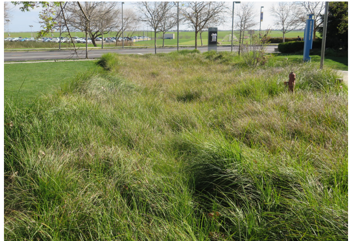
Stormwater can be detained in large swales or low-lying landscaped areas that are designed to receive and infiltrate stormwater during heavy rain events or flash flooding.
