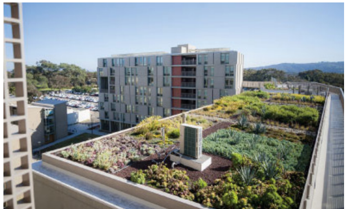
Keeling Apartments showcases a green roof.
