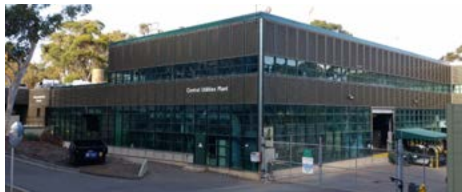
Central Utilities Plant.
