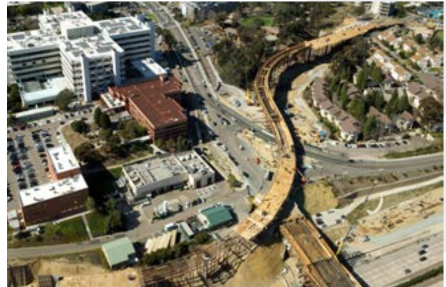
Gilman Bridge and Light Rail under construction.
