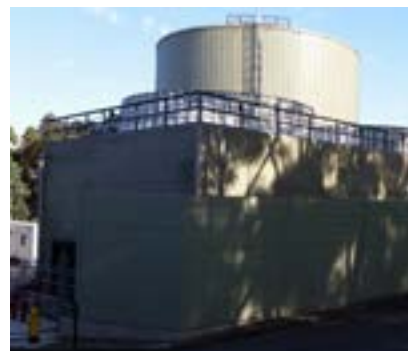
West Campus Cooling Tower.
