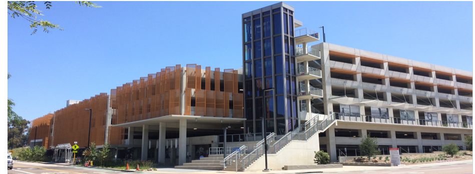
Athena Parking Structure on East Campus.
