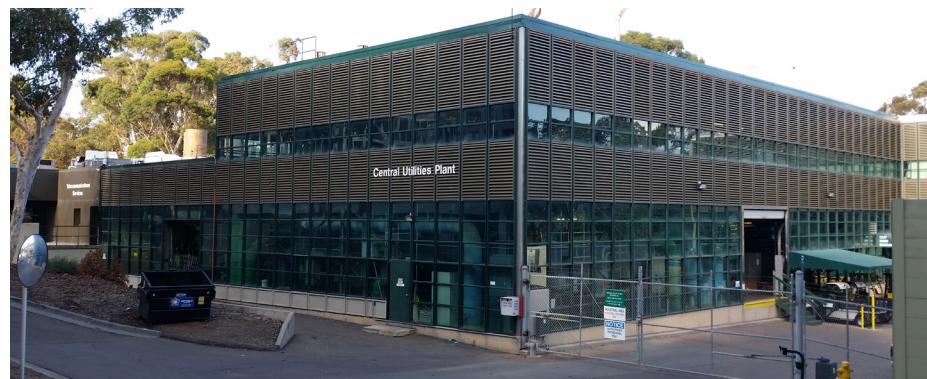
Central Utilities Plant.
