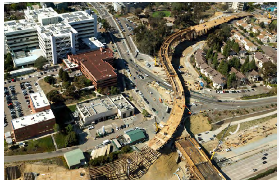
Gilman Bridge and Light Rail under construction.
