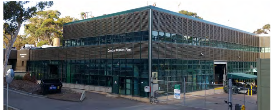
Central Utilities Plant.
