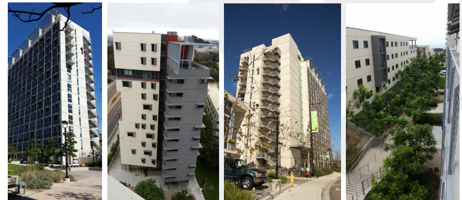
The Village Towers student housing, various views.
