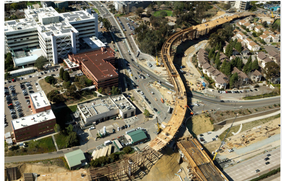
Gilman Bridge and Light Rail under construction.
