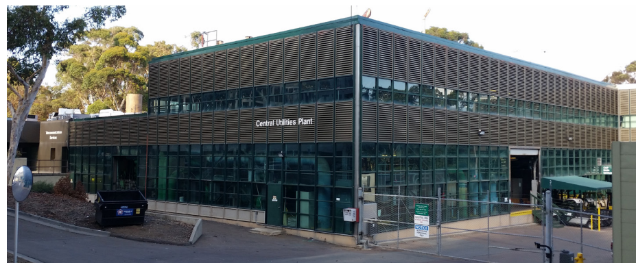
Central Utilities Plant.
