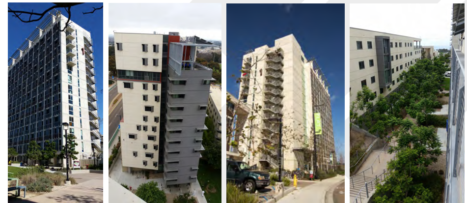
The Village Towers student housing, various views.
