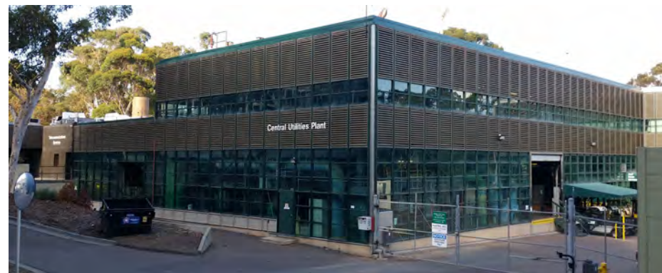
Central Utilities Plant.
