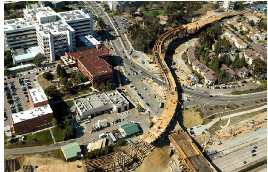
Gilman Bridge and Light Rail under construction.
