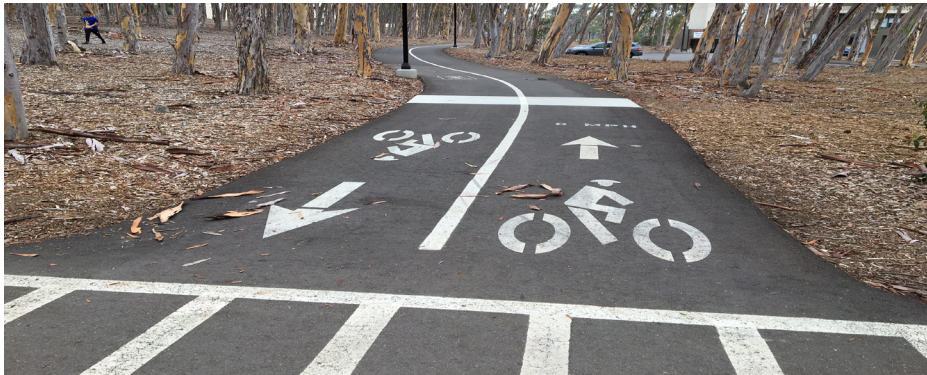
Dedicated bicycle and pedestrian path improvements.
