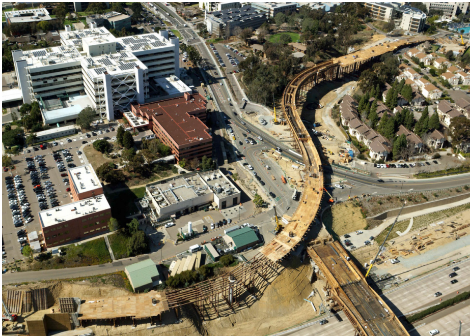
Gilman Bridge and Light Rail under construction.
