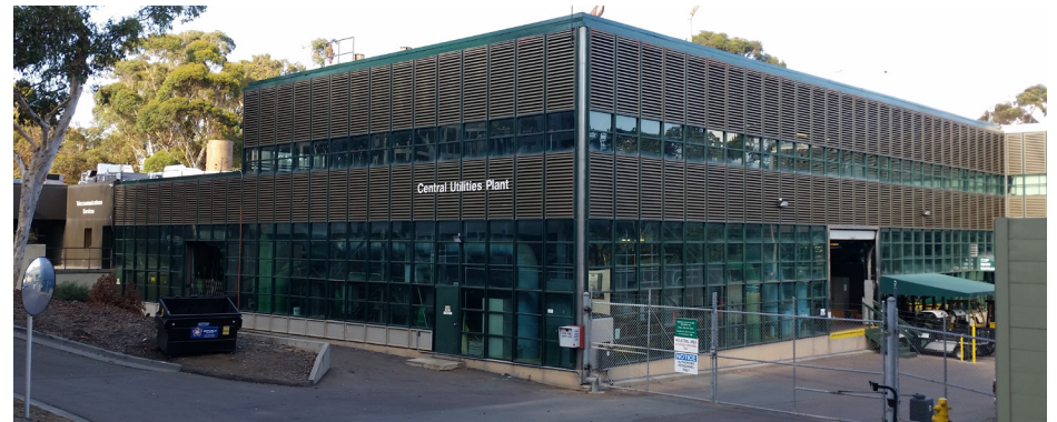
Central Utilities Plant.
