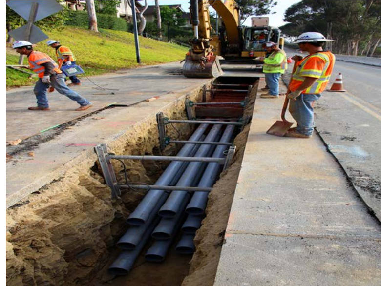
New duct bank on North Gilman
