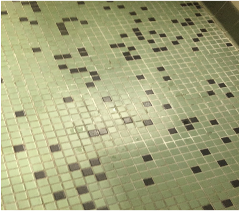
Restroom tile floor before
