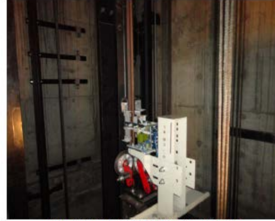
New roller guides and landing system all cars
