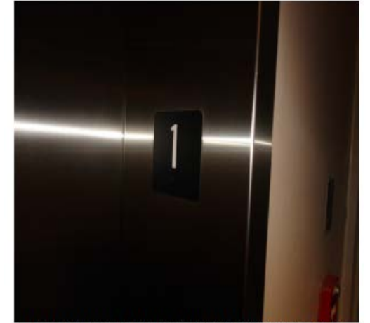
New code compliant entrance jamb floor plates with braille
