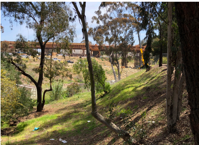
The guideway under construction in Pepper Canyon.
