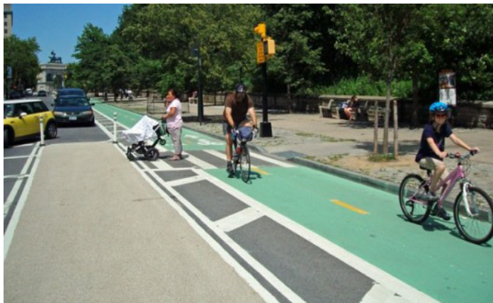
A two-way cycle track, as shown in Section C-Alternate, can provide safer passage for cyclists and a buffer for pedestrians.
