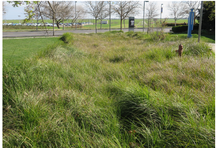
Stormwater can be detained in large swales or low-lying landscaped areas that are designed to receive and infiltrate stormwater during heavy rain events or flash flooding.
